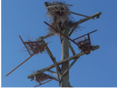
A close-up of the artificial structure from which nest platforms imitating tree branches jut out from the utility pole used to anchor the framework.
