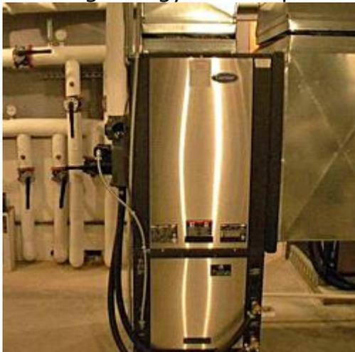
Among other energy use features, the Navarino Wildlife Center has a closed loop heating and air conditioning system consisting of a series of tubing buried under ground at water
