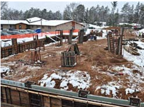
As with life in the northwoods, weather doesn't stop building construction.
