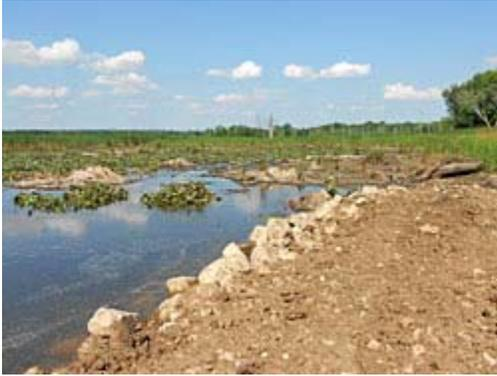
A crew pushed dirt and rock into place to stop the flow of water, resulting in an increase in the water level of about six inches.
