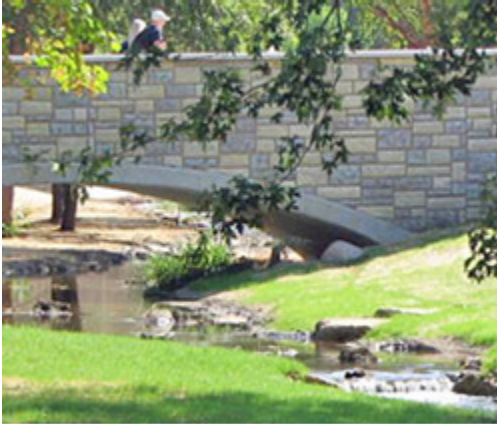
Restored stream with grass just starting to grow back along the banks. DNR Photo
