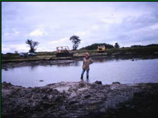
Plugging ditches, breaking tile at the Brooklyn Wildlife Area.
